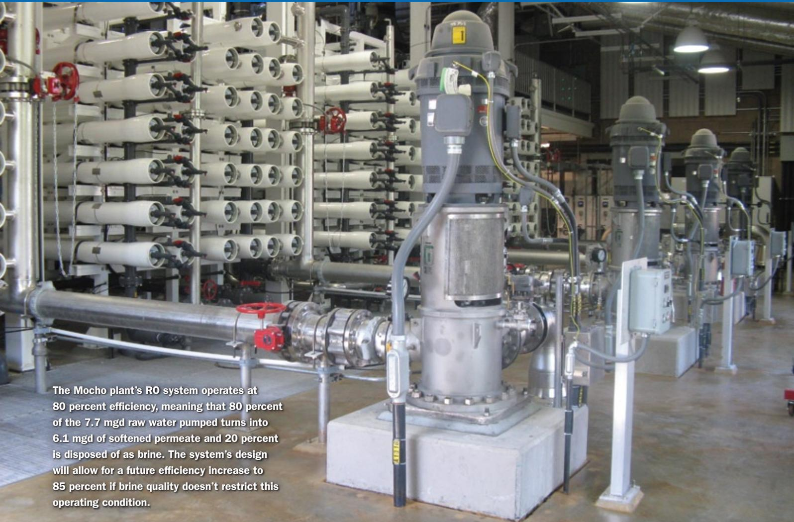
The Mocho plant's RO system operates at 80 percent efficiency, meaning that 80 percent of the 7.7 mgd raw water pumped turns into 6.1 mgd of softened permeate and 20 percent is disposed of as brine. The system's design will allow for a future efficiency increase to 85 percent if brine quality doesn't restrict this operating condition.
